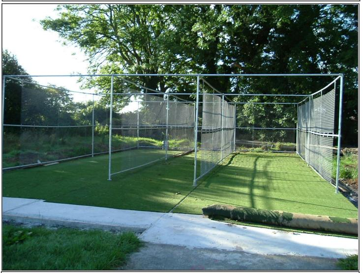
Due to the versatility of the Interclamp product range many structures can be produced using them in many differing and diverse industries. Here interclamps have been used for the construction of the frame for a 3 lane cricket practice enclosure. Interclamp have also been used for the construction and assembly of goal posts frames. Interclamps are a product range that can be sold across many market sectors
